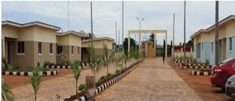
Plate 1: Entrance view of Federal Housing Estate Asaba (Fieldwork, 2023)
